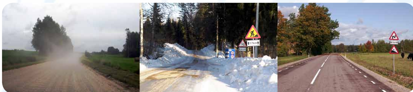
Road before reconstruction
